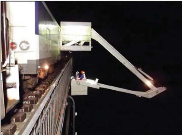
Figure 6. Inspection using hydraulic cradles
