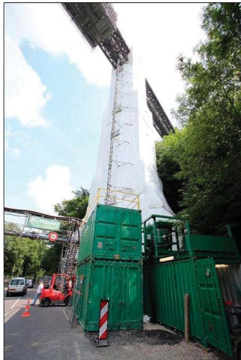
Figure 9. Sanding machines and abrasive tank containers
